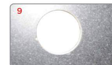
8 DRILLING TAP HOLE 9 Invert the Sink, Use the marking to Drill the Hole with Wood Cutting Bit
